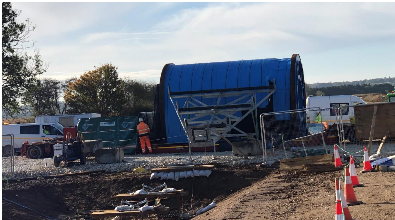
Figure 4.5: Cable Drum Delivered to Site
